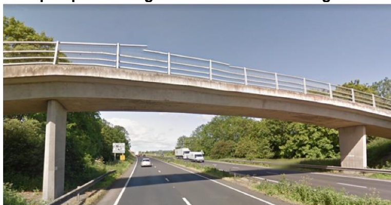
Figure 3.11: Current parapets on Higher Farm Lane overbridge
