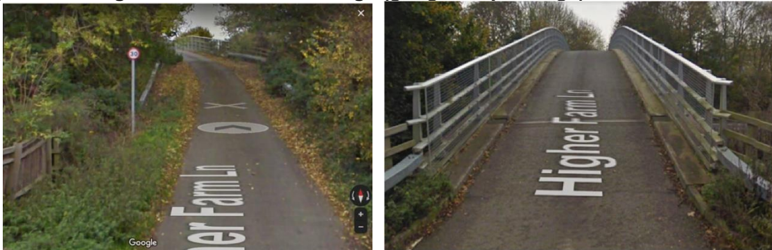
Figure 3.10: Higher Farm Lane overbridge (google maps image)
